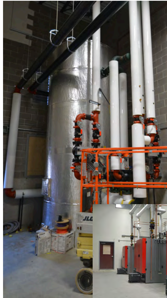
4000 gallon ASME tank, site insulated
