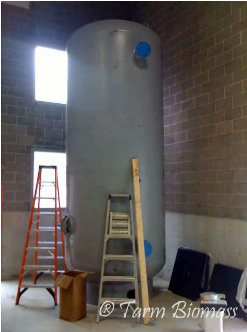
4000 gallon ASME tank, site insulated
